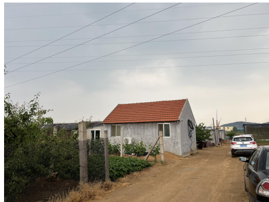
图2-8 110kV泽崮线#107~#108/110kV银白线#79~#80线路北侧17m, 四甲村西侧种植看护房
